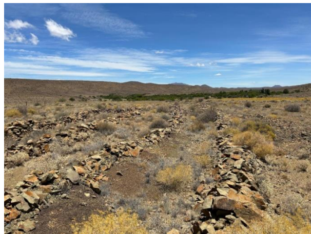
Erosion/flood control measures (low rock berms) on site
